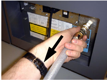
Figure 14: Disconnecting air supply
