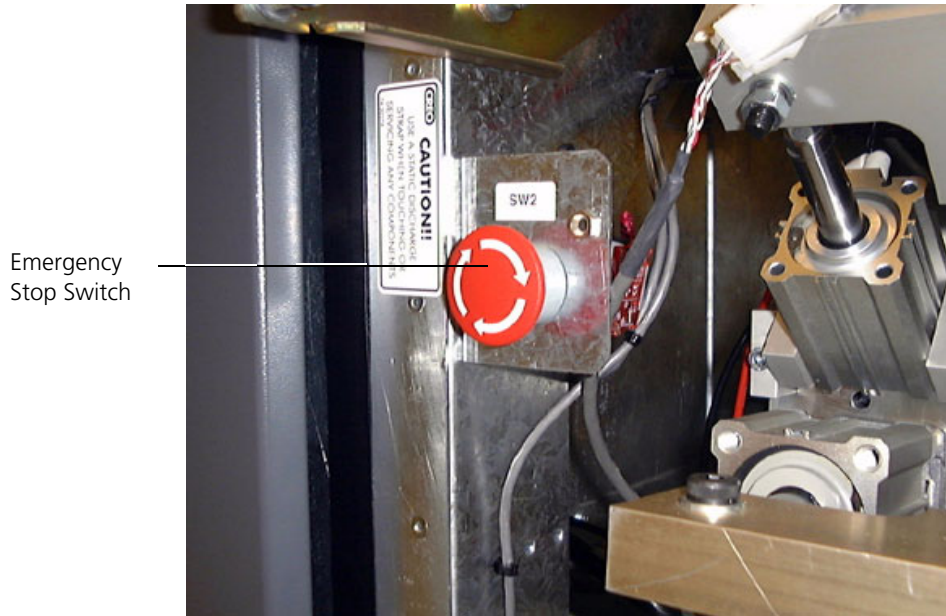
Figure 4: Emergency Stop switch
